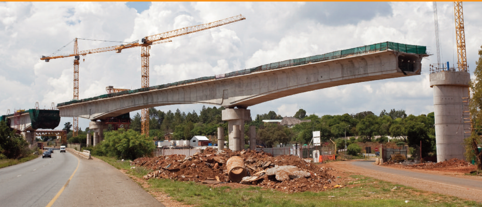
Gautrain construction, South Africa. iStock/Getty Images
